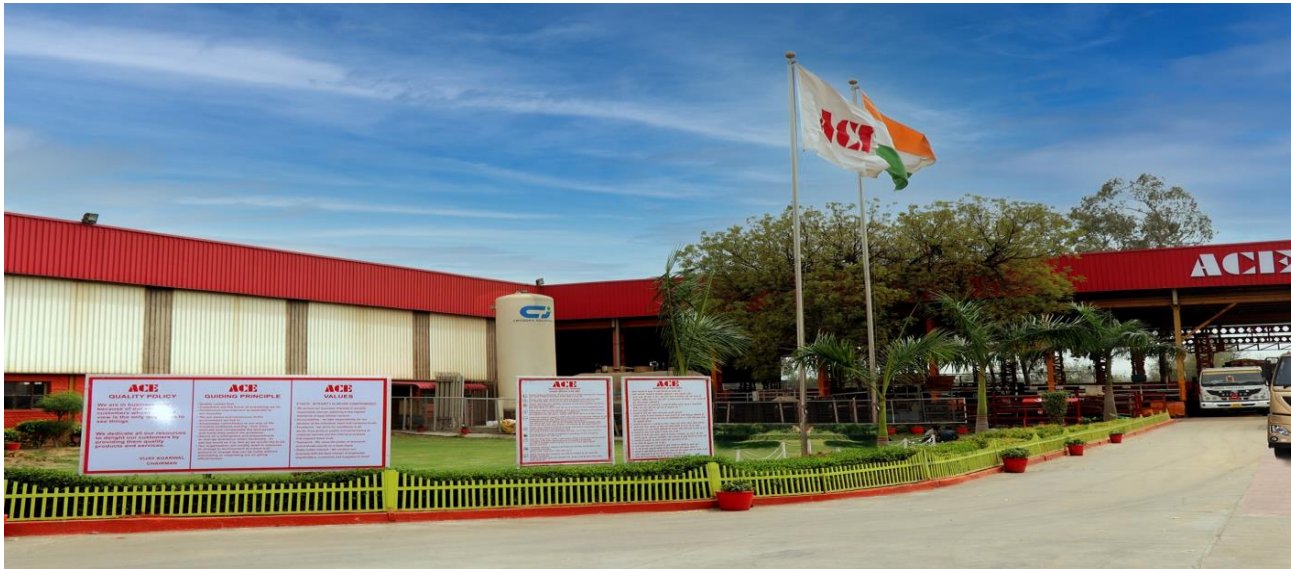
Fabrication Unit and Weld Shop
